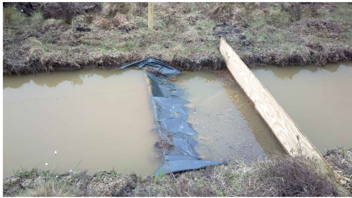
Baffle/Weir Detail
