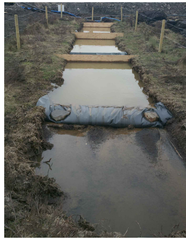
Completed Settling Pond System
